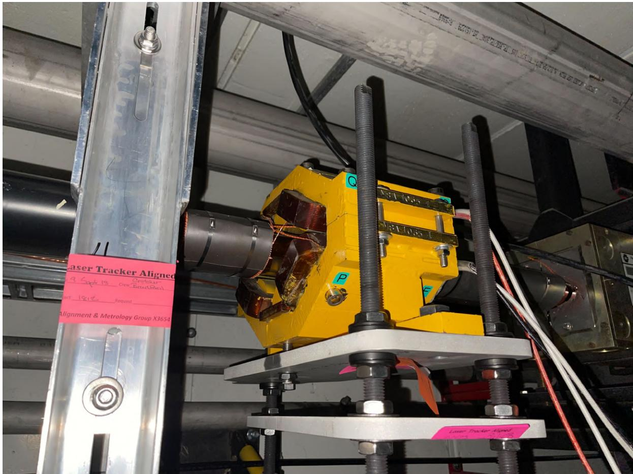
Figure 7.2 Newly installed compensation sextupoles in the 620 section.
